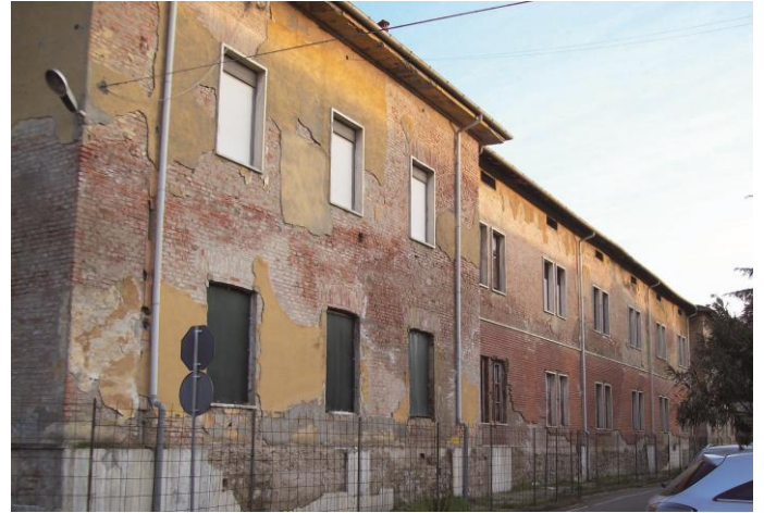
Figure 1. External front of the strategic building of Pistoia.
